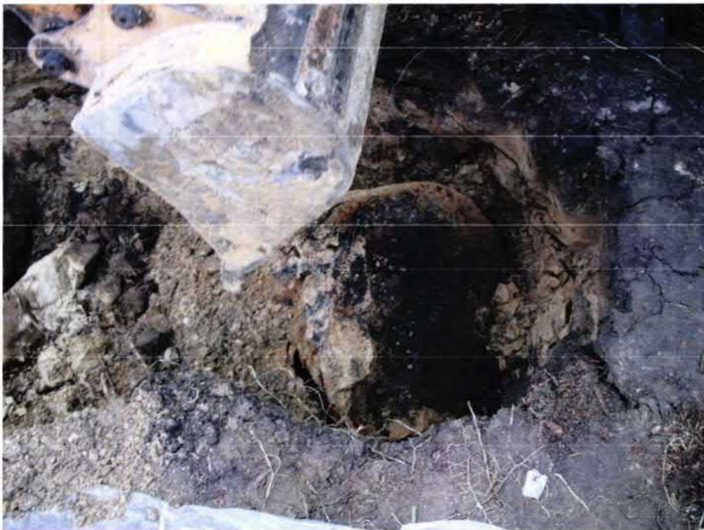
Picture 2: UST 729Bluebell during removal.
